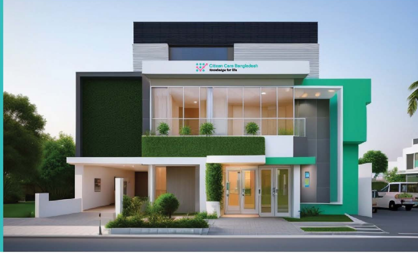
3 Storey Citizen Care Building
